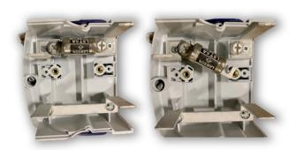
Lawson Type "LST" fuse-links are for use in single-phase street lighting cut-outs or similar installations. These fuse-links comply with UK Electricity Supply Industry Standards and BS7654.
